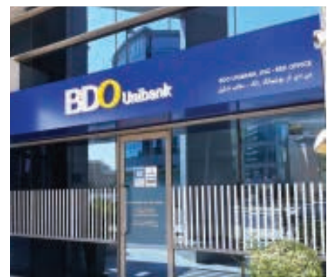
The new BDO office in Dubai
